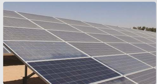
Figure 2. Soiling, such as dust, on PV modules reduces power output.
